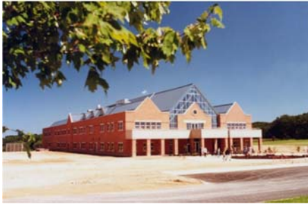
Washington Road Campus opened with the Great Hall and Classroom Building C in 1990.
