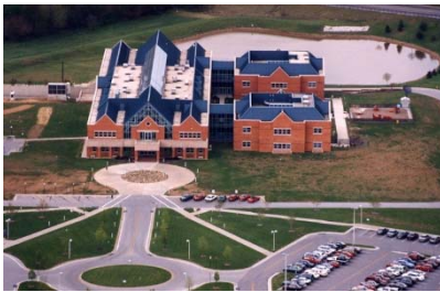
Multipurpose Building M, funded entirely by Carroll County, opened in 1993.
